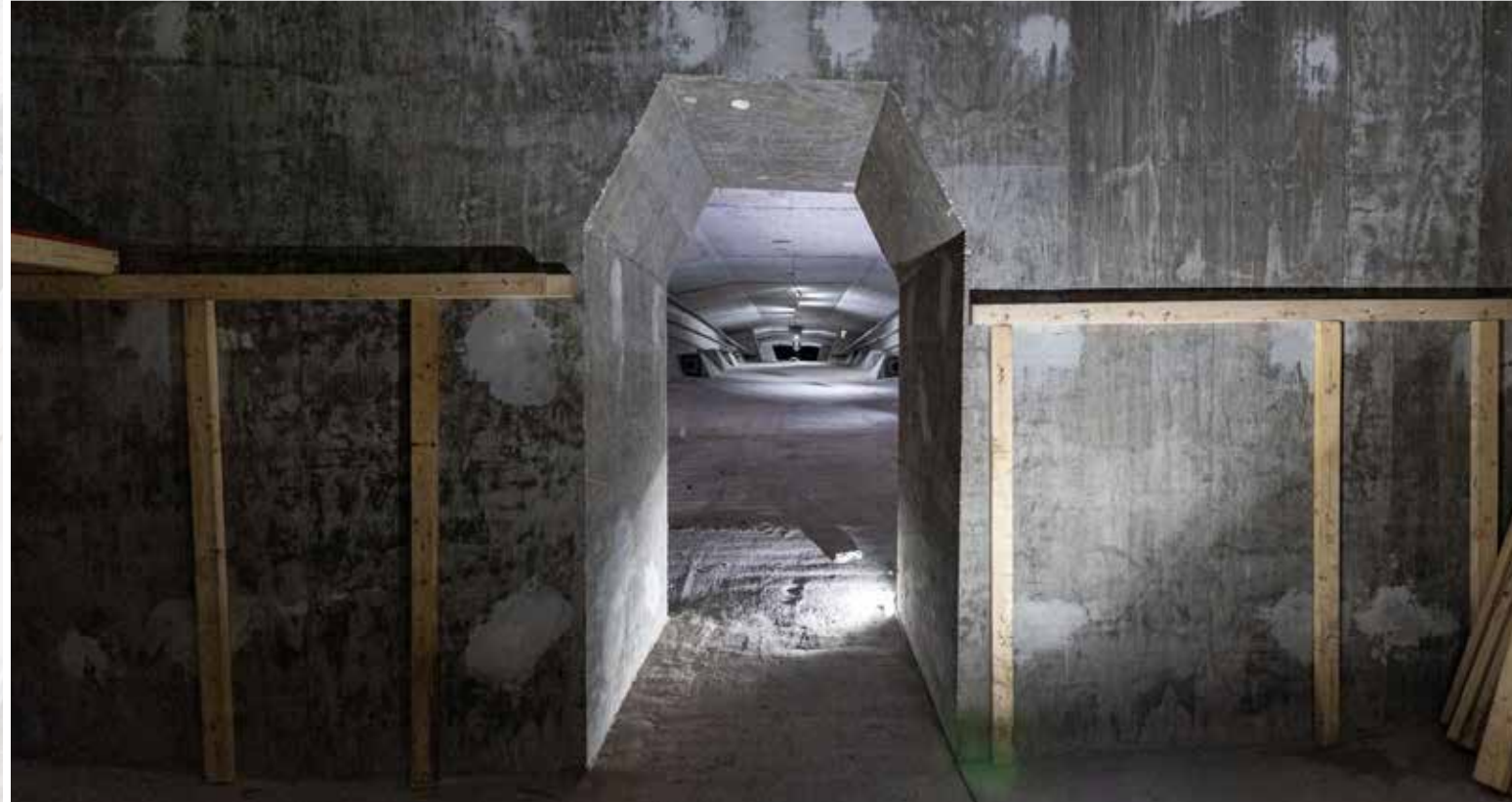
Segmental Bridge – Interior Box
