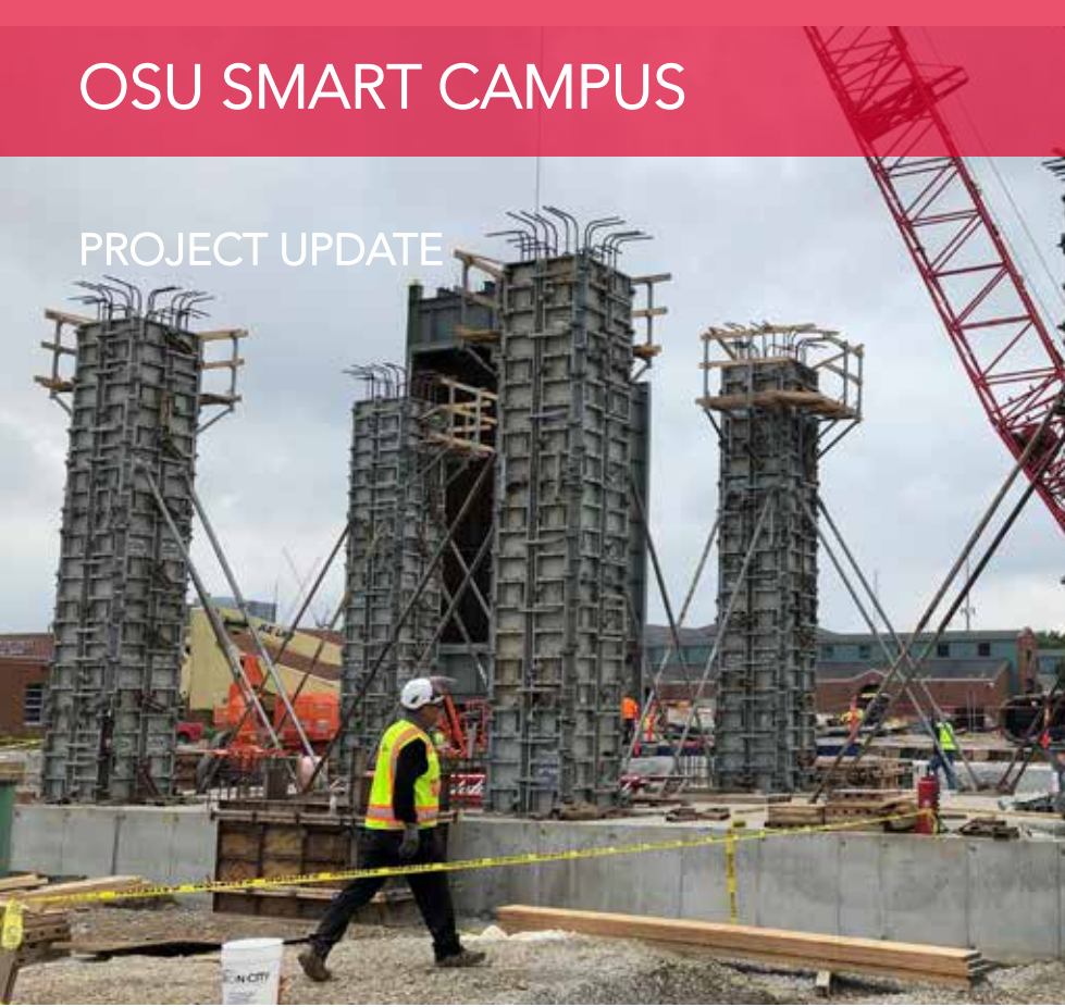
Pumping Concrete for Steam Turbine Generator Columns
