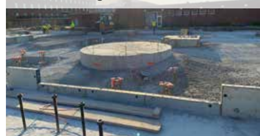
Backfilling for Slab on Grade
