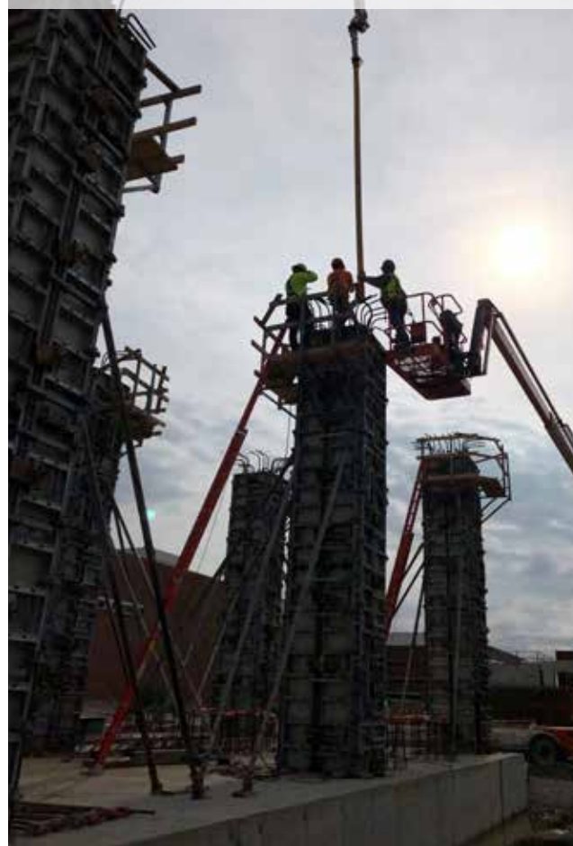
Pumping Concrete for Steam Turbine Generator Columns
