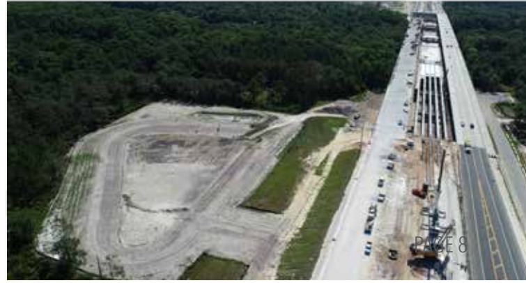
Wekiva River Segmental Bridge
