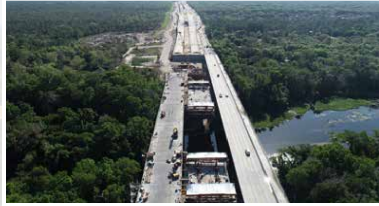
Wekiva River Segmental Bridge
