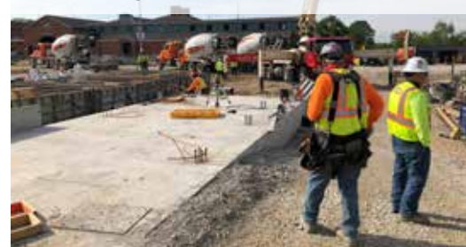
Backfilling for Slab on Grade
